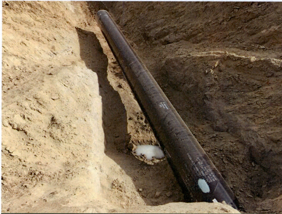
Report Photo #1 "Milky Water Seep Beneath County Road 7 HDD Pipe":
